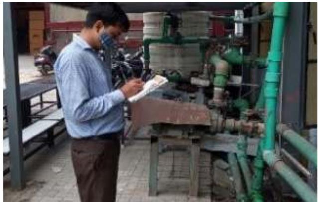
Soccer International Pvt. Ltd., a Jalandhar based MSME, manufactures sports goods since 1976. As a part of our project, a walk-through energy audit was conducted, and it was identified that the electricity consumption at the unit was not optimized. By repairing the power factor controller, the unit is now saving over INR 20,000 per month and conserving 200044 kwh of electricity in a year.
