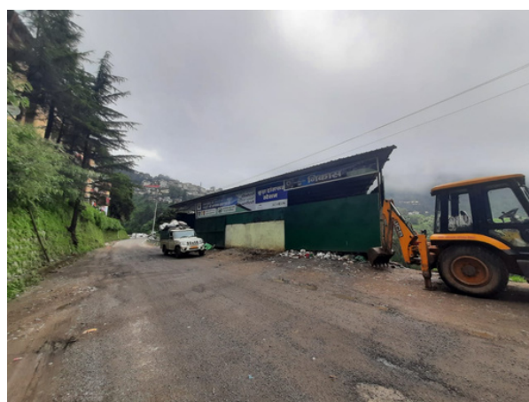
Photos of the field visit to Mussori project
